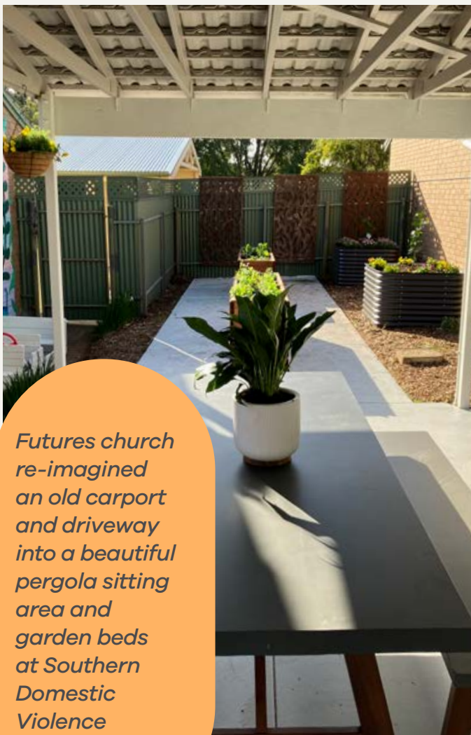
Area at SADVS prior to renovation to a new pergola sitting area for clients and staff.
